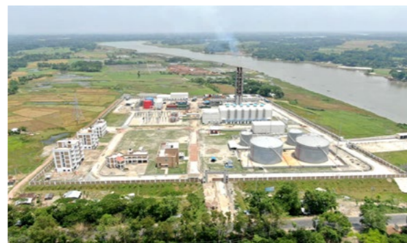
The Genertec CMC Madhumati heavy oil project in Bangladesh created a green plant area and monitored the production and domestic sewage in real time to ensure that the sewage met the discharge standard.
