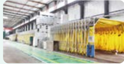
VOCs treatment implemented by Genertec Shenyang Machine Tool
