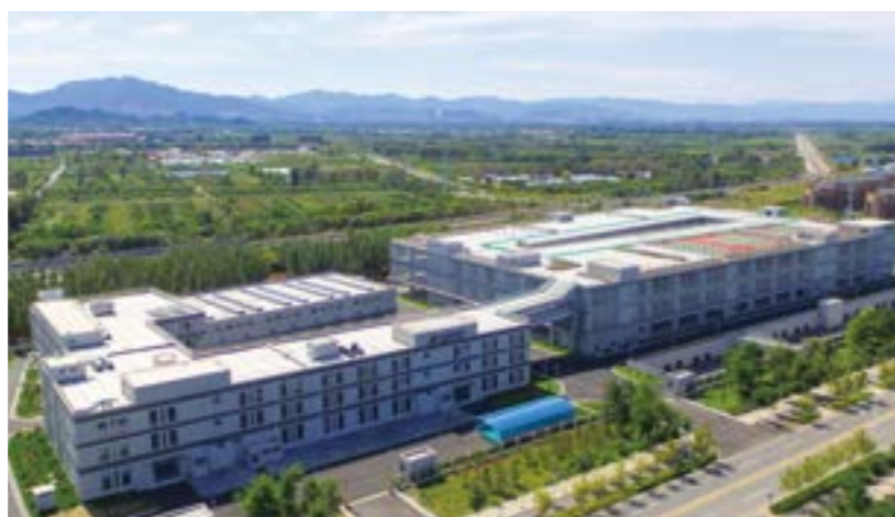
Key supporting project of the Winter Olympics – Yanqing Comprehensive Transportation Service Center undertaken by Genertec Xinxing
