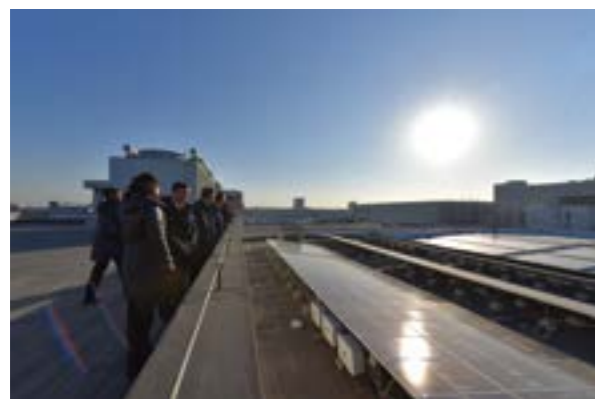
Photovoltaic power generation project undertaken by Beijing Precision Machinery & Engineering Research Co., Ltd., which is affiliated to Genertec Machine Tool Engineering Research Institute Co.,Ltd., a subsidiary of Genertec Machine Tool, was completed with the installed capacity of 1.8MW and average annual power generation of 1.907 million kWh
